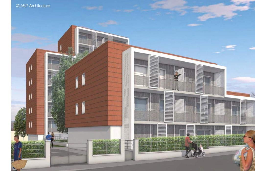
**The Jules Ferry residence** of the social housing provider Le Toit Vosgien in Saint-Dié-les-Vosges (88) is currently the highest straw-insulated building (7 floors). Seven hundred prefabricated caissons filled with straw were used on the site.
