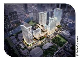
The complex will incorporate an architectural system known as the Climate Ribbon™, devised by Swire Properties. It is a trellis composed of steel, fabric and glass which will connect the buildings together. It will span 14,000 m<sup>2</sup> of the exterior part of the shopping centre.
