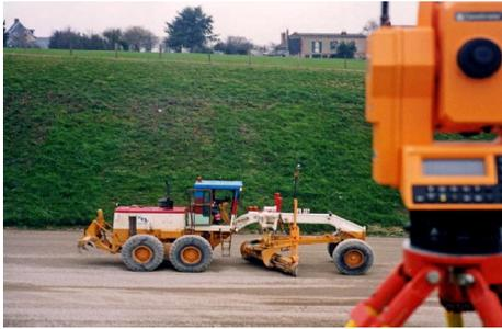
Earthmoving is a vital prerequisite to the start of large road or rail infrastructure projects, for example. The performance of earthmoving contractors depends largely on their ability to use plant to grade layers of materials as regularly as possible so as to facilitate the placement of blacktop or rails. DTP Terrassement, a Bouygues Construction subsidiary, is using an innovation implementing satellite navigation systems to guide earthmoving plant.
