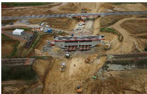
Bouygues Construction designed and built the 125-km-long stretch of the A28 motorway between Rouen and Alençon in a record time of 48 months. In order to reduce disturbance to infrastructure crossed by the new road, Quille, a Bouygues Construction subsidiary, developed a new procedure for placing overpasses which is known as “Transpra”.
