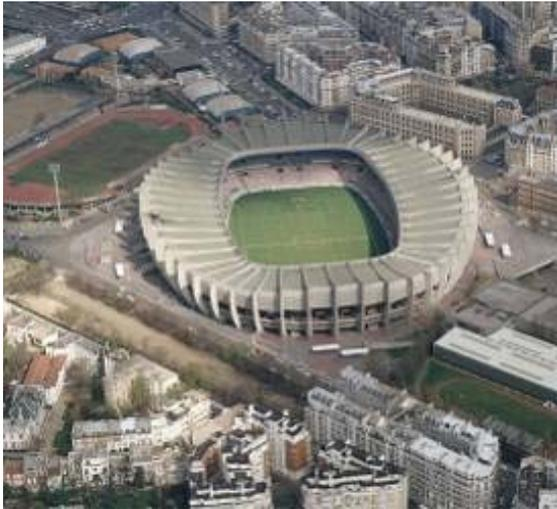
The construction of the stadium required the installation of a giant elliptical shell assembled from precast concrete segments. Assembled on-site with the use of synthetic resins, they were installed with prestressing.
