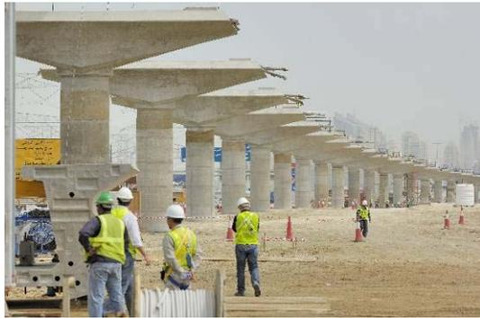
VSL, the Bouygues Construction subsidiary specialising in post-tensioning and cable-stay bridges, carried out the construction work on the Red Line, the elevated metro line crossing Dubai. In a joint venture with Freyssinet International and Rizzani de Eccher, VSL precast 13,000 voussoirs for the viaduct and erected them over a distance of 45 km, using eight launching girders.
