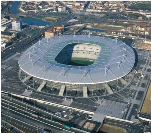
Design, construction, operation and maintenance of a stadium with 80,000 covered seats and a total of 36,000 m<sup>2</sup> of net usable surface. Built on a 14-hectare site, the Stade de France features an elliptical disk-shaped roof suspended 42 metres above the pitch. The playing surface is sunk below natural ground level, reducing the external height of the imposing stadium.
