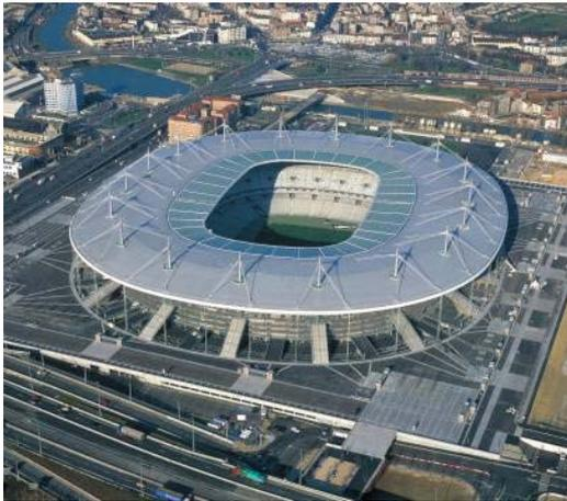
Design, construction, operation and maintenance of a stadium with 80,000 covered seats and a total of 36,000 m<sup>2</sup> of net usable surface. Built on a 14-hectare site, the Stade de France features an elliptical disk-shaped roof suspended 42 metres above the pitch. The playing surface is sunk below natural ground level, reducing the external height of the imposing stadium.
