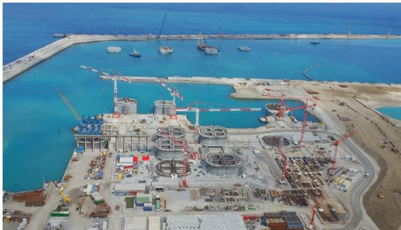
Tanger Med II port: mass prefabrication of 105 5,000-tonne caissons
